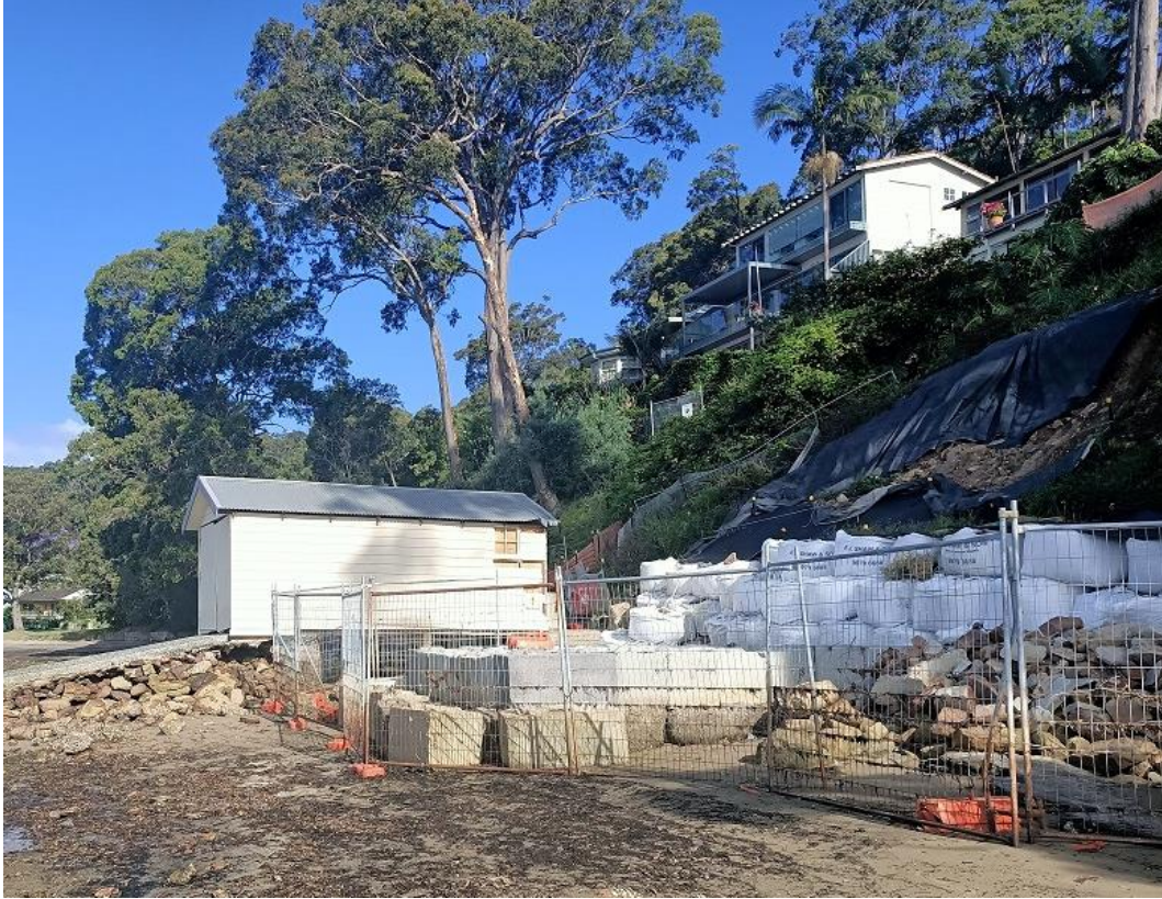
Figure 2 Temporary structure and work platform following seawall collapse.
