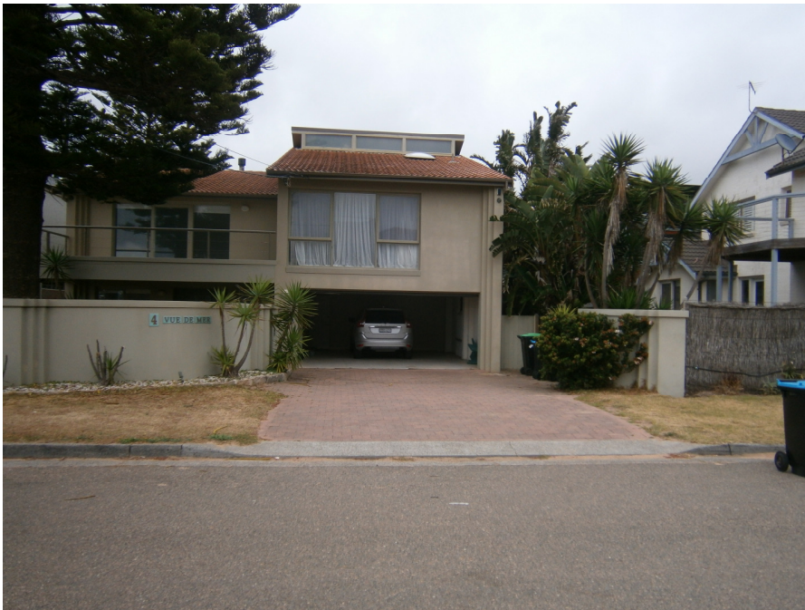
Existing Residence as viewed from Loftus Road
