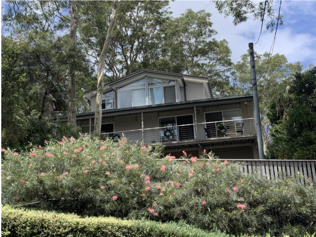
Fig 3: View of subject dwelling, looking south-east from Wandeen Road
