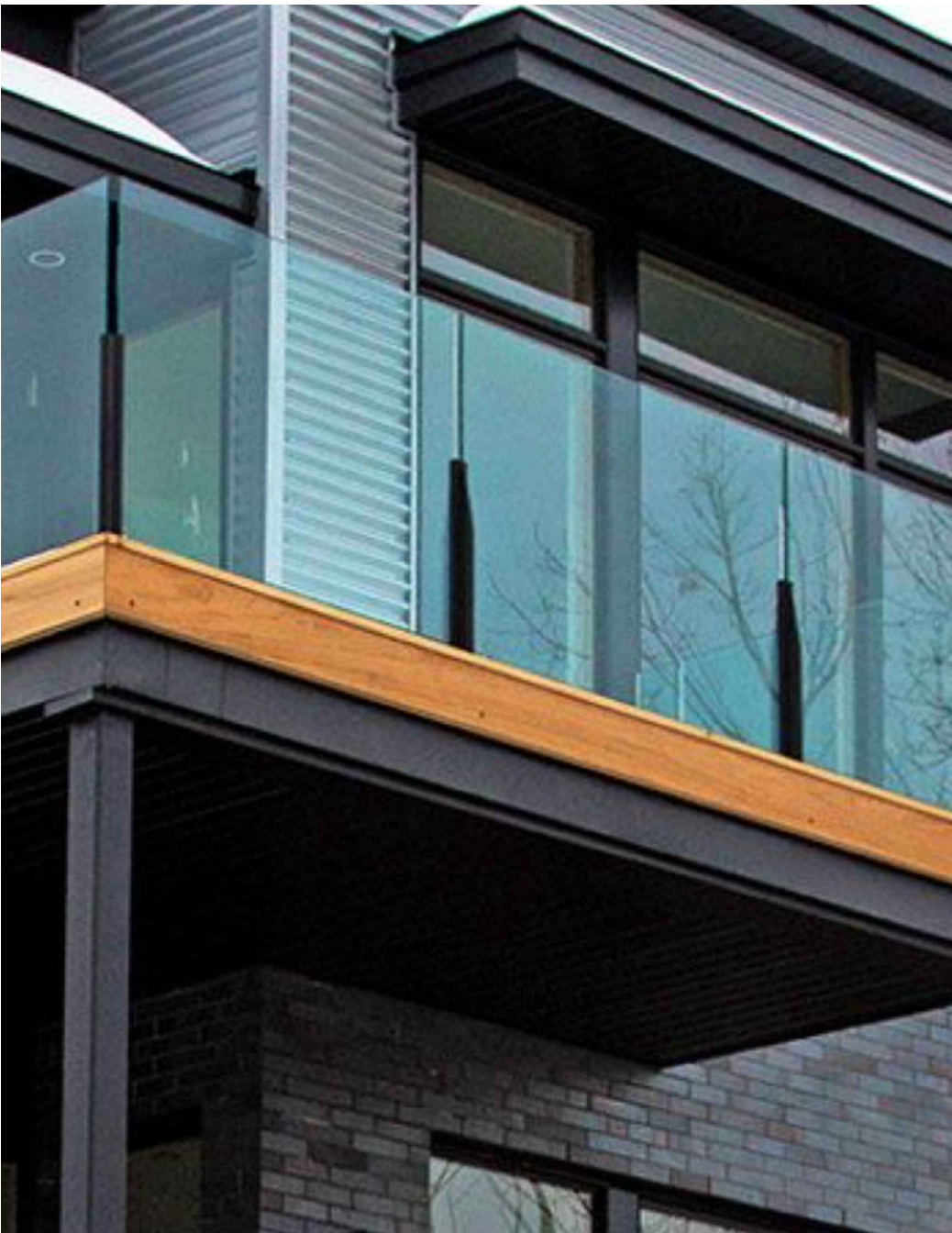
BLACK ALUMINUM BALUSTRADE SUPPORT - 15.5 LAMINATED SAFETY GLASS
