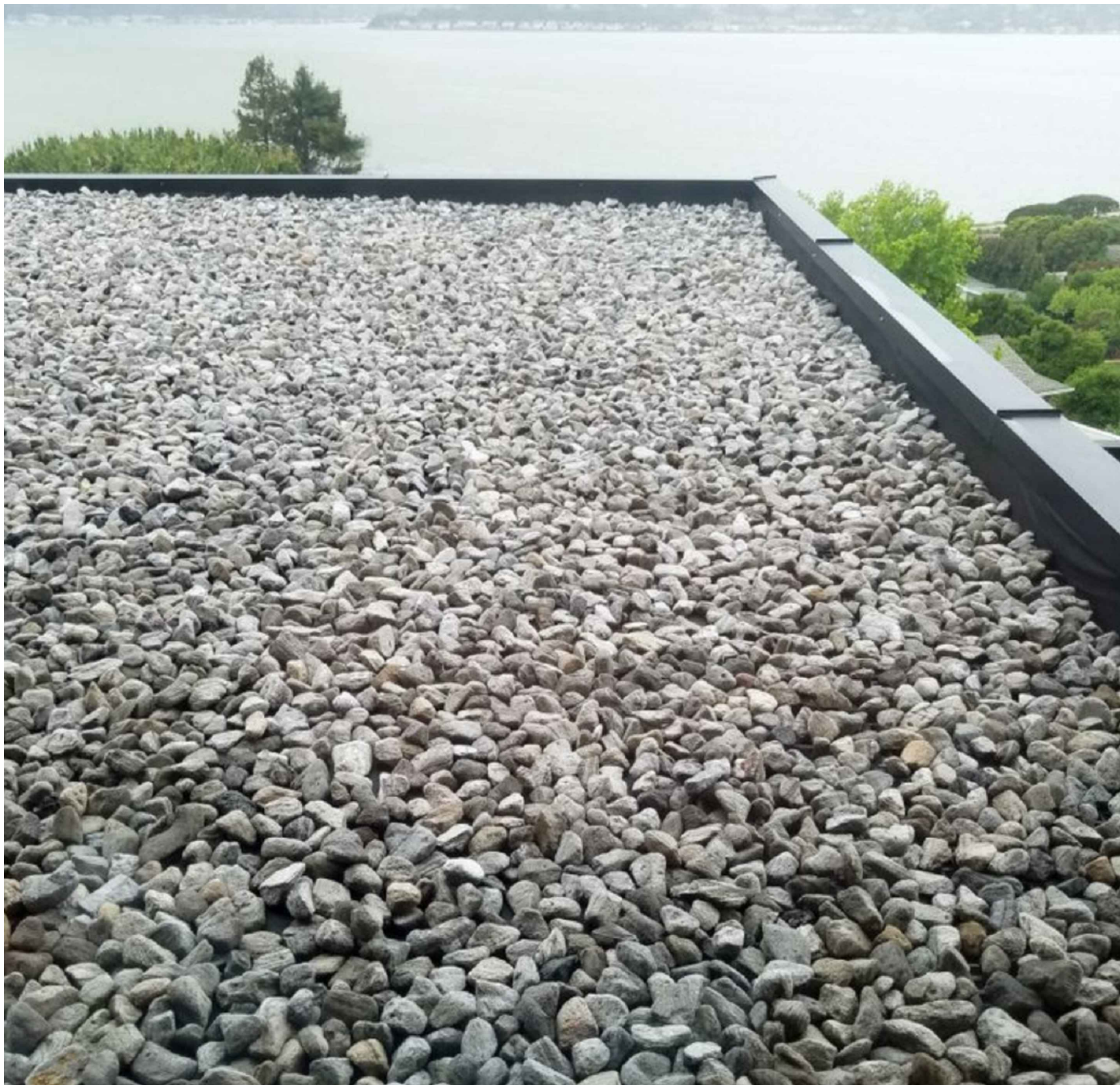
RIVER GRAVEL BALLAST ROOF WITH SAFETY MESH - BIRD PROOF
