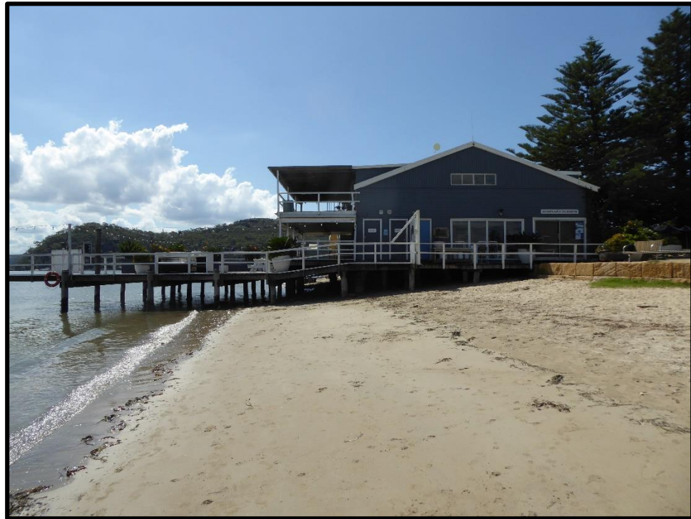
EXISTING BUILDING VIEWED FROM THE SOUTH
