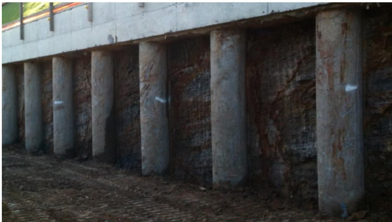
Plate 1: Photograph of Soldier Pile Wall Prior to being Shotcreted (Figure 3 from Witt Report)
