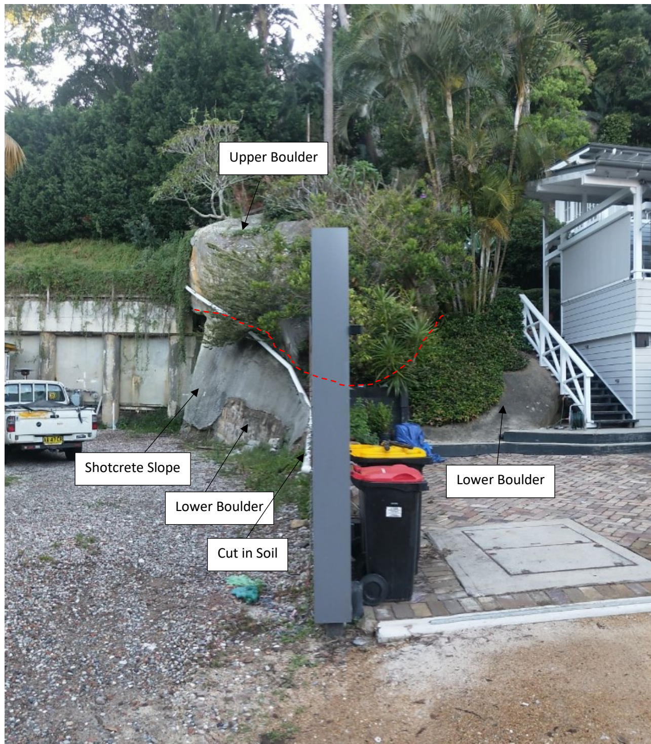
Plate 3: Photograph 2 of Large Boulders and Shotcreted Cut Face At/Near Southern Boundary (Facing East)
