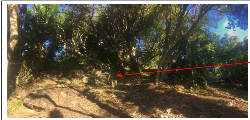
Rough Sandstone Boulder Wall
