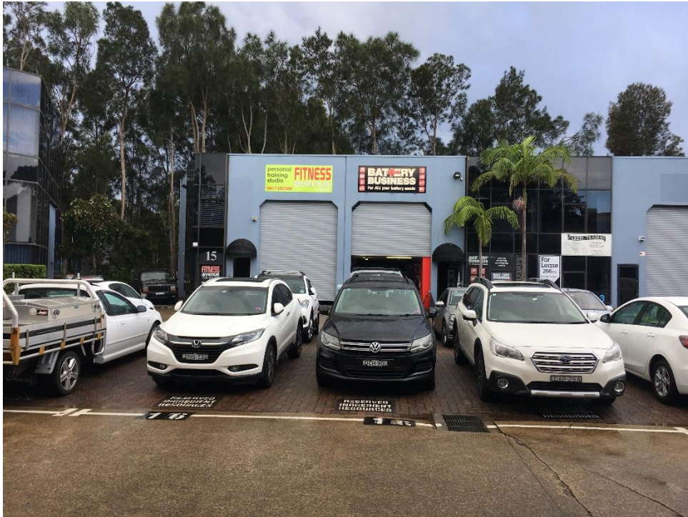
Photograph 3 View of the existing property looking south
