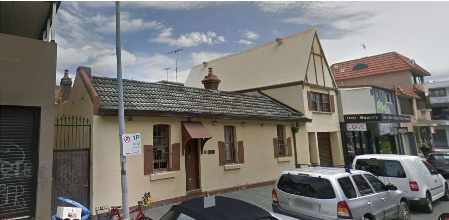
EXISTING COTTAGE ELEVATION
