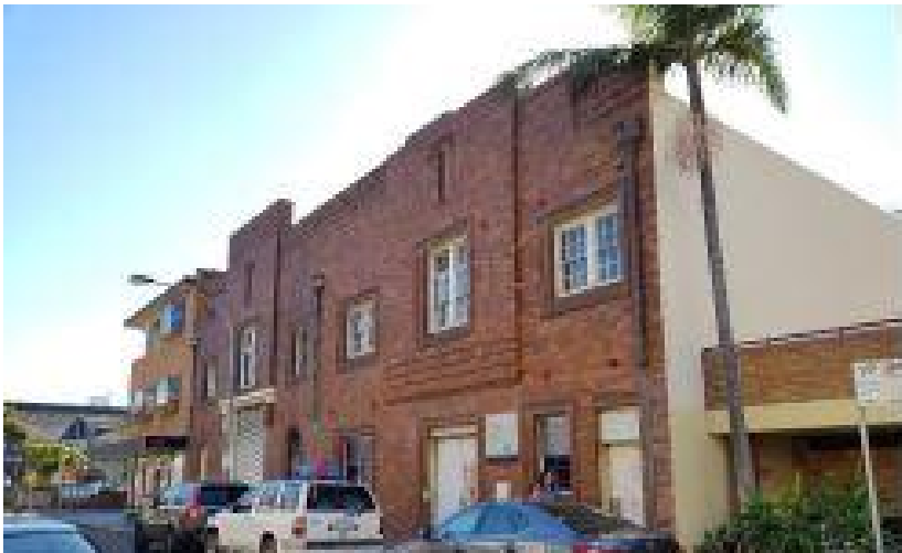
No.33 MANLY SUBSTATION
