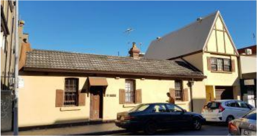
EXISTING COTTAGE ON SITE 21 WHISTLER STREET
