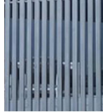
BS3 - ALUMINIUM BATTEN SCREEN TYPE 03, TO MATCH DULUX "SHALE GREY" OR SIMILAR
