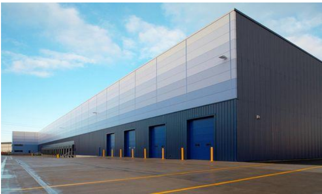
Precast concrete tilt panels with combined Kingspan/Danpalon cladding to roof height.
