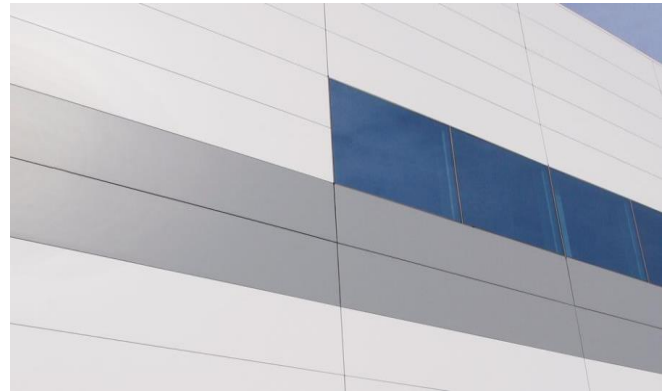
Precast concrete tilt panels with combined Kingspan/Danpalon cladding to roof height.
