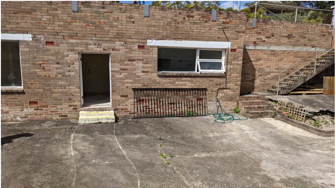
Photograph 4: Observation of minor cracks on concrete at the back of building.
