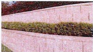
Sandstone block retaining wall example.
