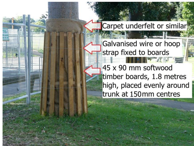
Figure 3 – Detail of Trunk Protection
