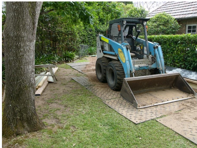
Figure 4 – Showing typical detail for truck mats.
