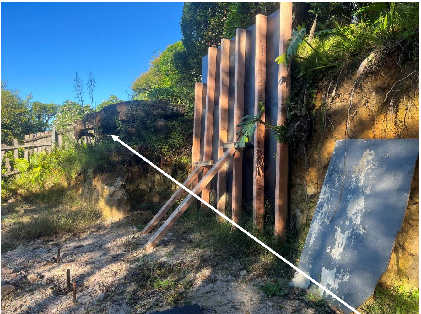
Rear of site showing cut that requires a higher retaining wall to retain higher ground level and rock outcrop that is now unstable
