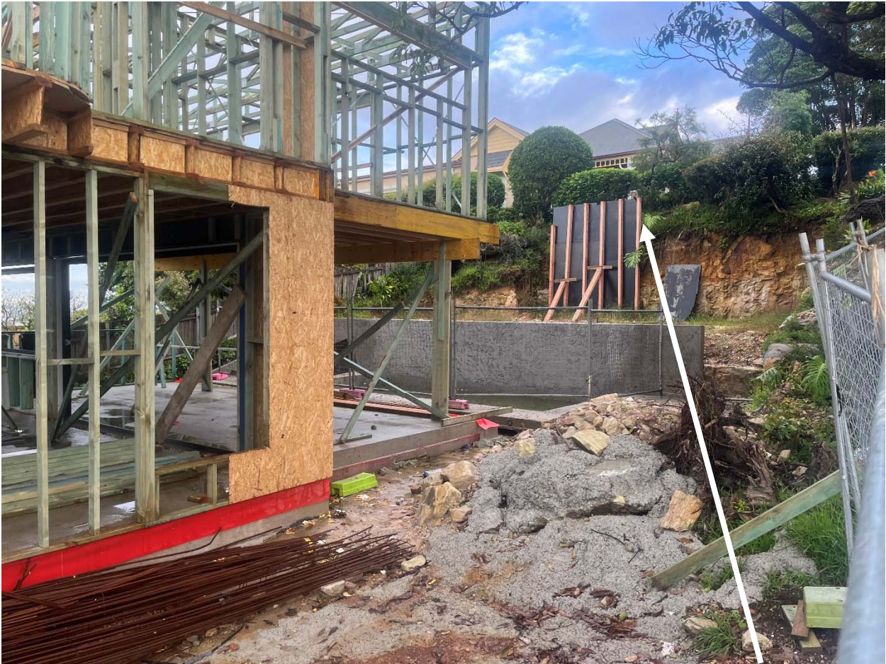
Rear of site showing existing cut that requires a higher retaining wall to retain higher ground level
