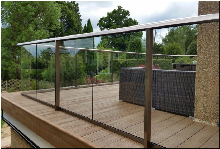
1. STAINLESS STEEL AND GLAZED BALUSTRADE
