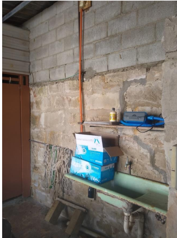
Photograph 3: Sandstone block wall
