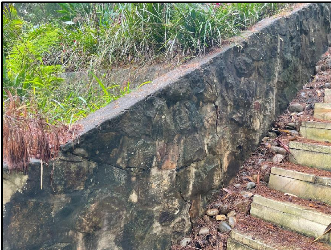
Photo 9 – View of typical sandstone rock wall with minor cracking.
