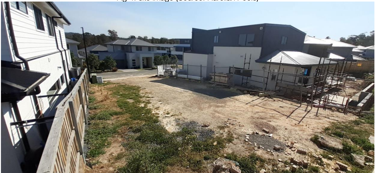
Fig 5: site image (Source: Narellan Pools)
