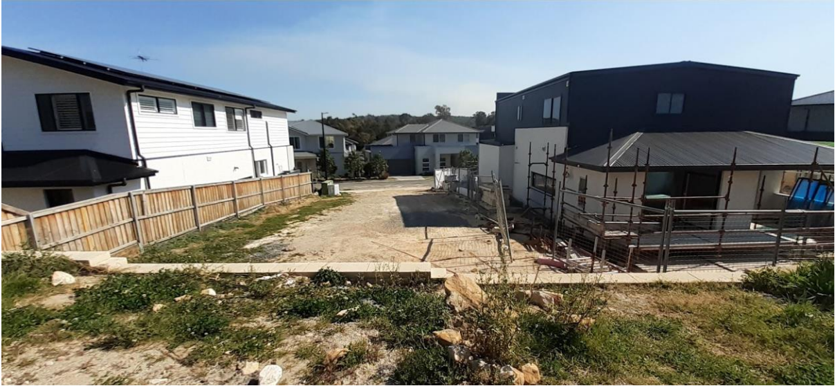
Fig 4: site image (Source: Narellan Pools)
