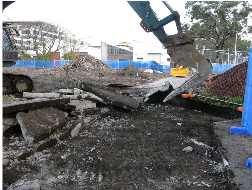
Figure 6 – Showing method for removal of concrete pavement, by carefully lifting sections and folding over the remaining paved surface.
