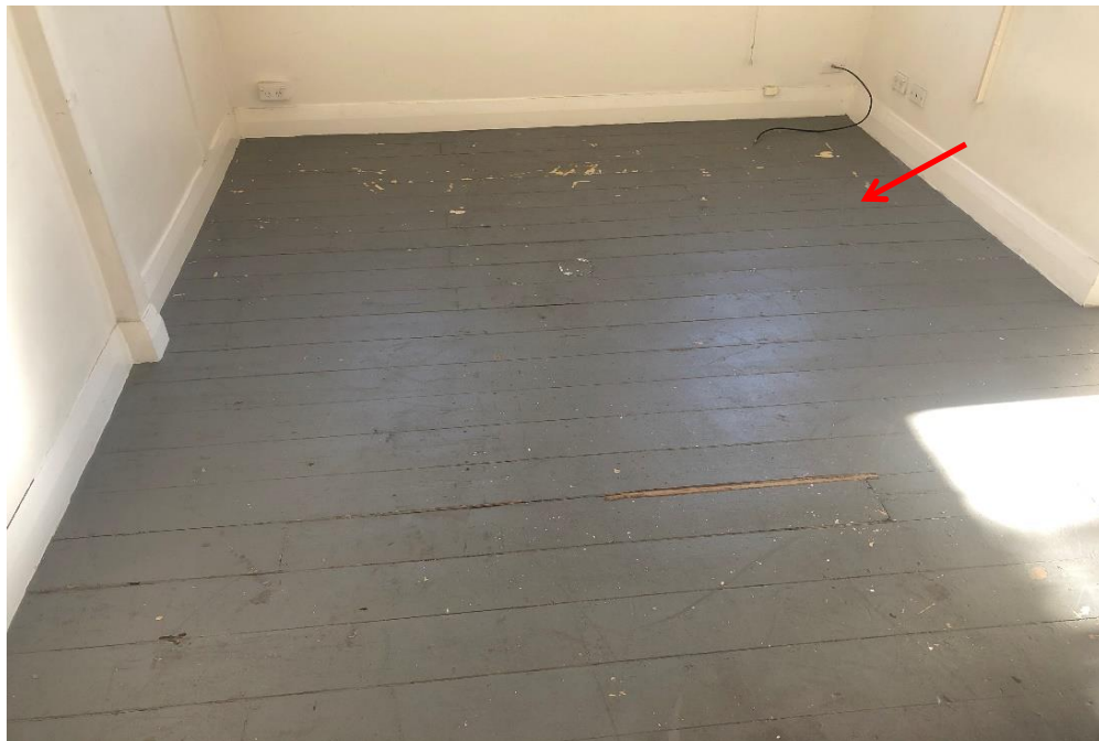
Photograph 20: 2 Dee Why Parade, Dee Why, internal, level 2, apartment 1 and 2, wall paint covering, throughout, typical white paint, non-lead paint ( \leq 0.1\% lead w/w)
