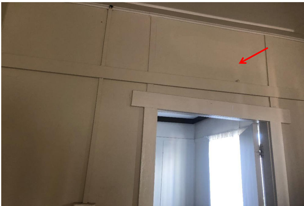
Photograph 26: 2 Dee Why Parade, Dee Why, internal, level 2, apartment 2, internal walls, paint covering, typical cream paint, non-lead paint ( \leq 0.1\% lead w/w)
