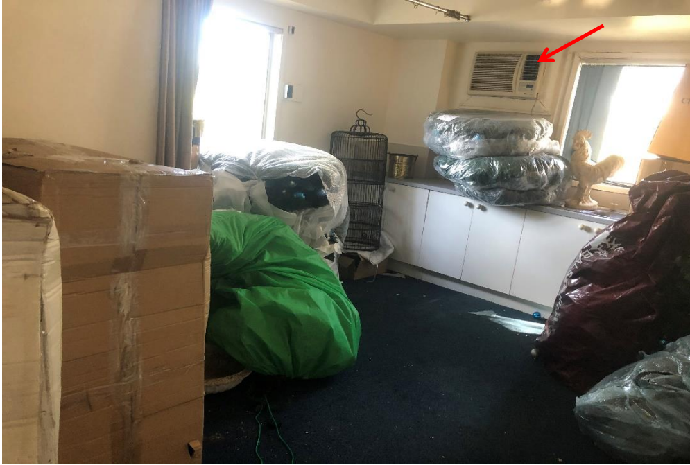
Photograph 29: 2 Dee Why Parade, Dee Why, internal, ground floor, A/C units, throughout, bulk internal insulation, suspected SMF.
