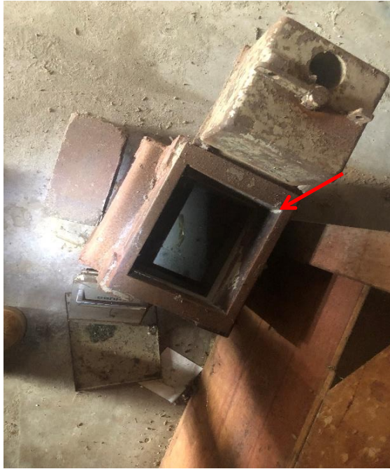
Photograph 33: 2 Dee Why Parade, Dee Why, internal, basement storage area, west elevation, chubb safety deposit box, safe lining, suspected non-asbestos.
