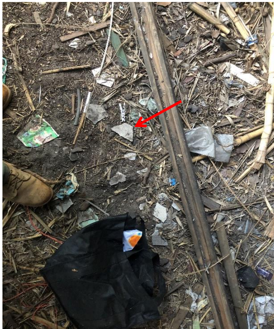
Photograph 10: 2 Dee Why Parade, Dee Why, external, eastern elevation, entrance to subfloor and throughout subfloor, ground debris, fibre cement sheeting, asbestos detected by analysis.
