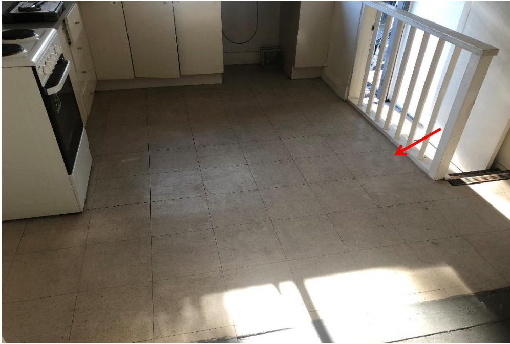
Photograph 19: 2 Dee Why Parade, Dee Why, internal, level 2, apartment 1 and 2, kitchen floor covering, beige dappled grey vinyl floor tile, no asbestos detected by analysis.
