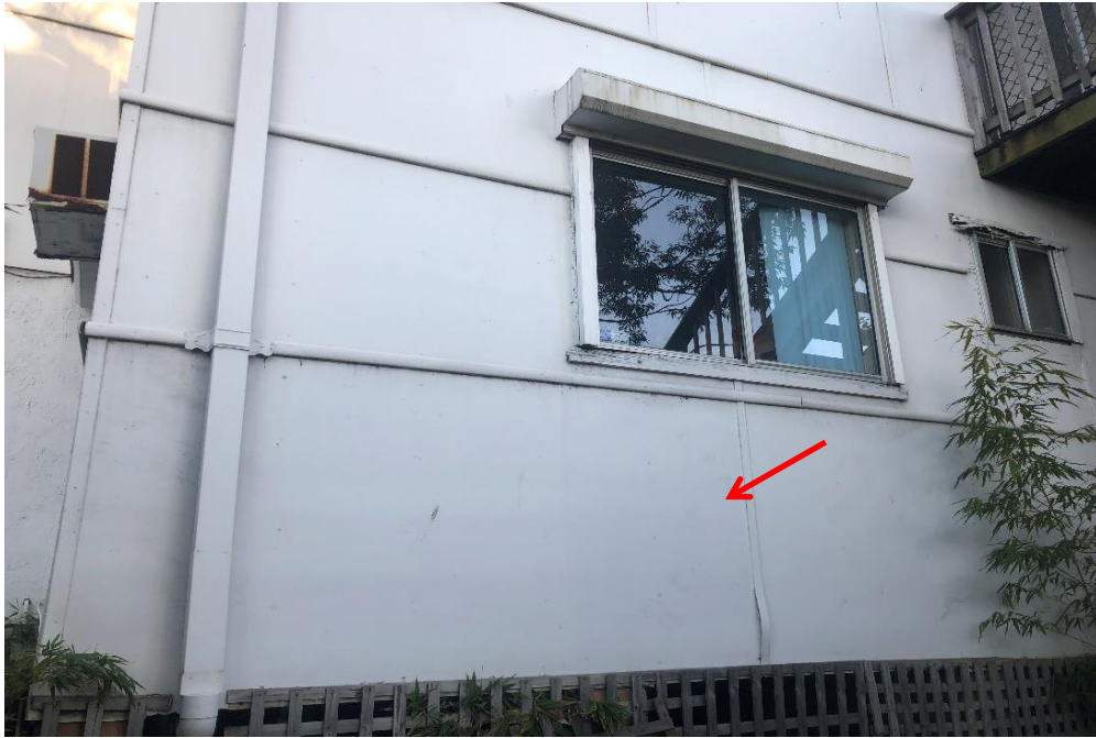
Photograph 9: 2 Dee Why Parade, Dee Why, external, throughout, wall material, fibre cement sheeting, no asbestos detected by analysis.
