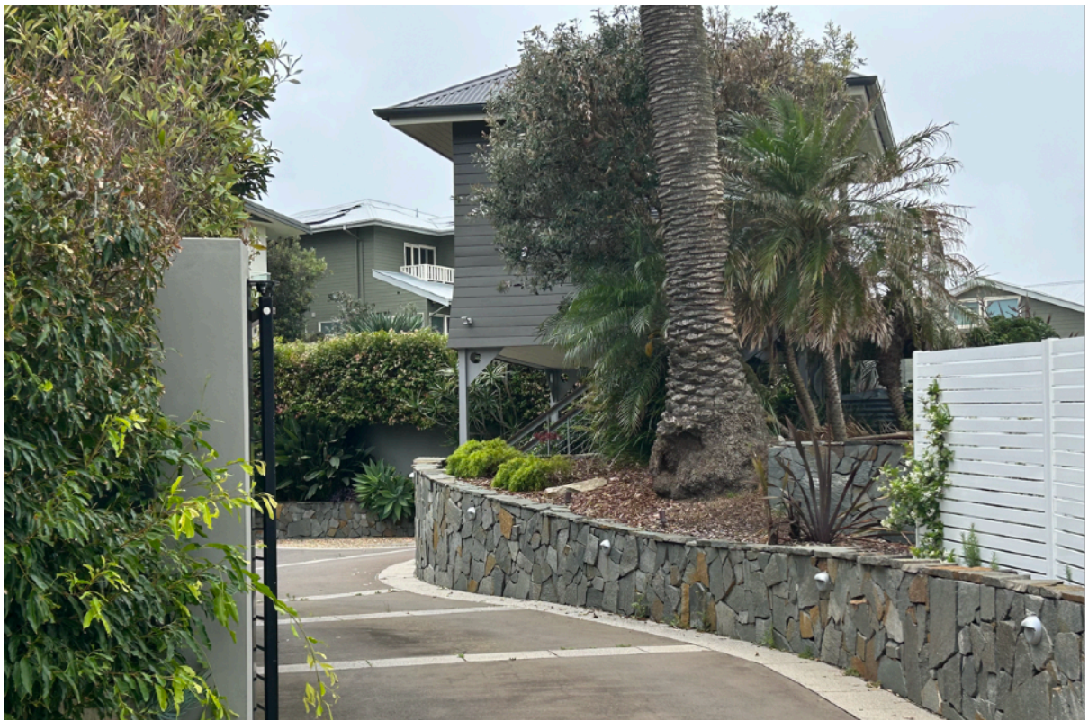
Figure 9: Beyond the Lillipilli hedge 81 Myola Road as viewed from the top of the shared driveway Source: Blackwattle Planning
