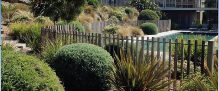
Regulation pool fencing concealed by shrubs and plantings with 900mm clearance from pool barrier
