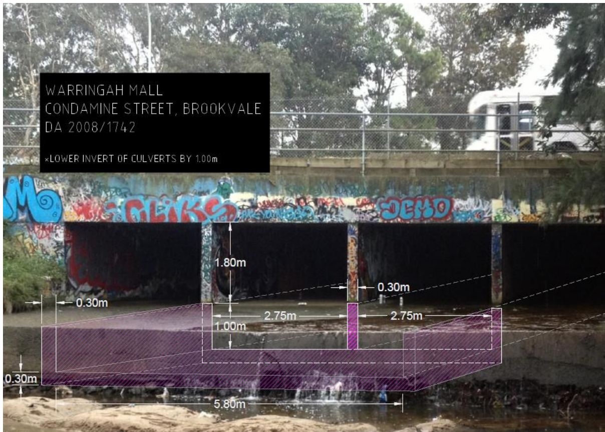
FIGURE 2 – PHOTOMONTAGE OF PROPOSED CULVERT WORKS
