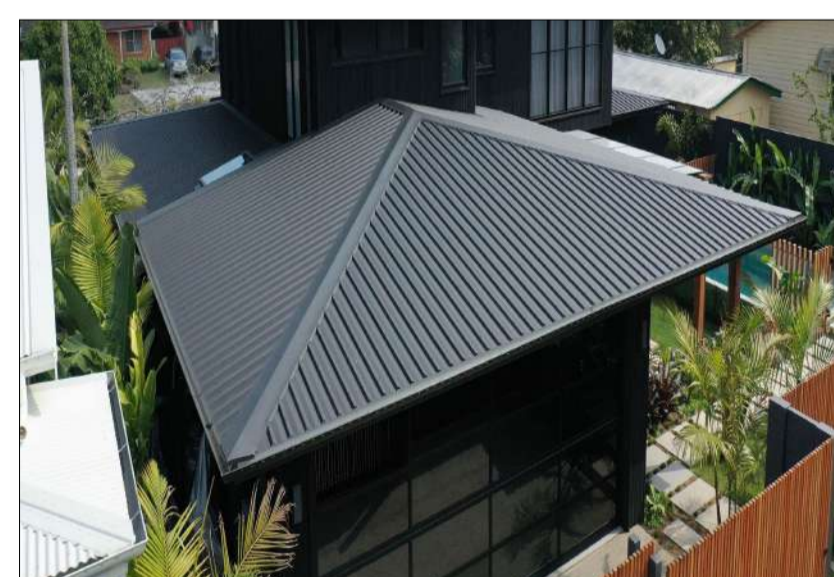
3. COLORBOND MONUMENT METAL ROOF
