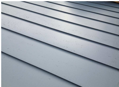
ROOF/CAPPINGS/ FLASHINGS/DOWNPipes: STANDING SEAM ZINC CLADDING
