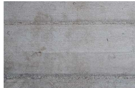
GARAGE/FIRST FLOOR WALLS: OFF-FORM CONCRETE
