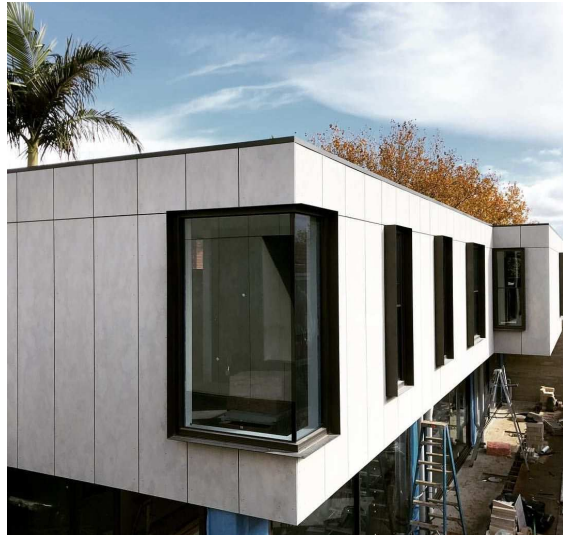
CLADDING/WINDOW FRAMES: CEMINTEL "BARESTONE" AND CHARCOAL/BLACK ALUMINIUM WINDOW FRAMES
