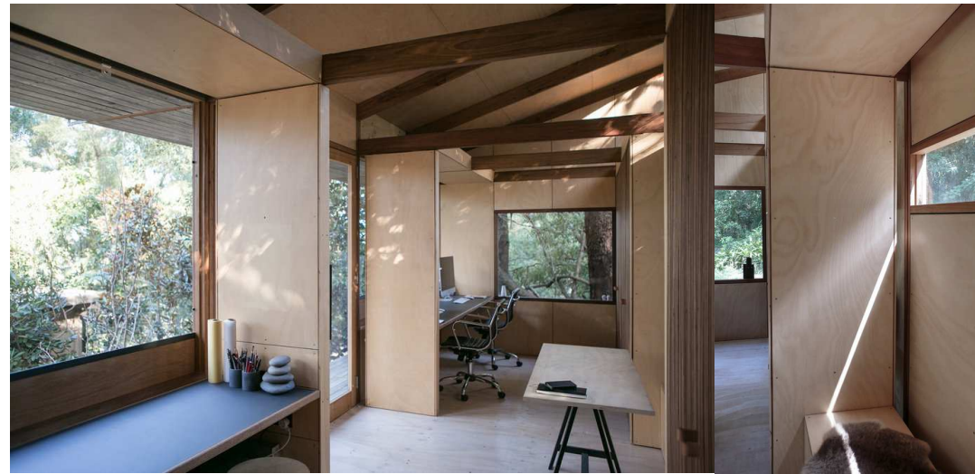
INTERNALS: PLY LINING HILIGHTS AND EXPOSED HARDWOOD FRAMING/HARDWOOD INTERNAL DOOR FRAMES.
