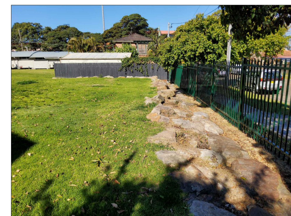
EXISTING ROCK RETAINING WALL ALONG SOUTHERN BOUNDARY TO BE REMOVED, FENCE TO BE RETAINED
