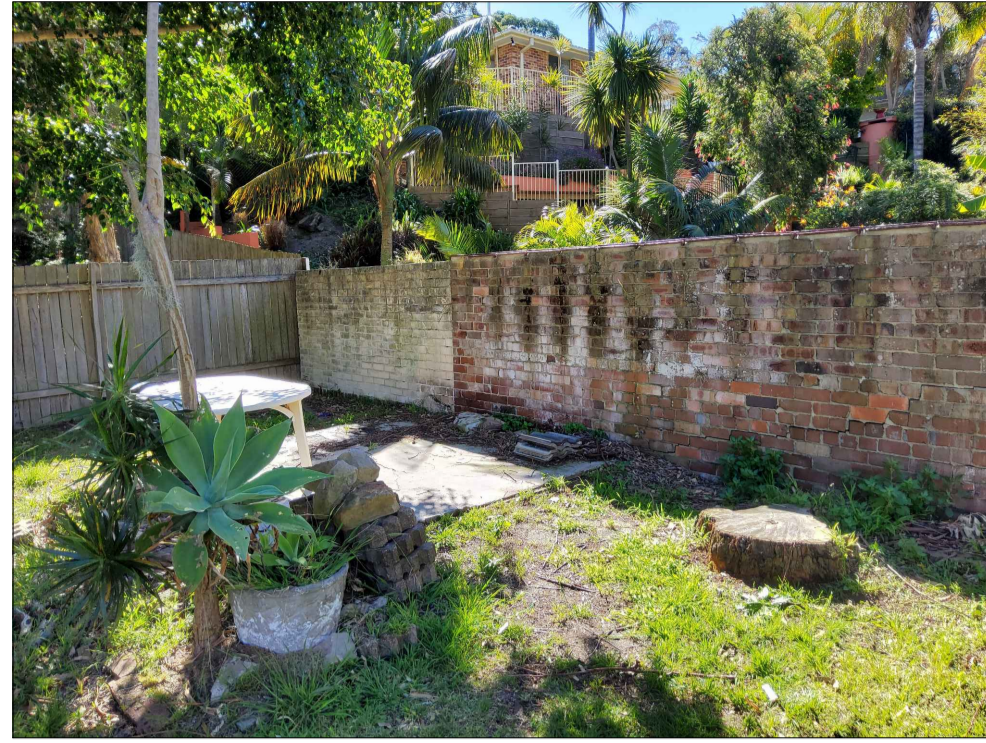
NORTHERN BOUNDARY NEAR COUNCIL DRAINAGE ASSET. MASONRY WALL TO BE RETAINED AND REPAIRED
