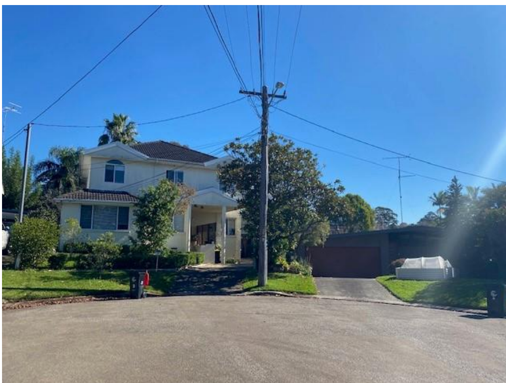
Photograph of 3 and 4 Bindi Place to the west of the site
