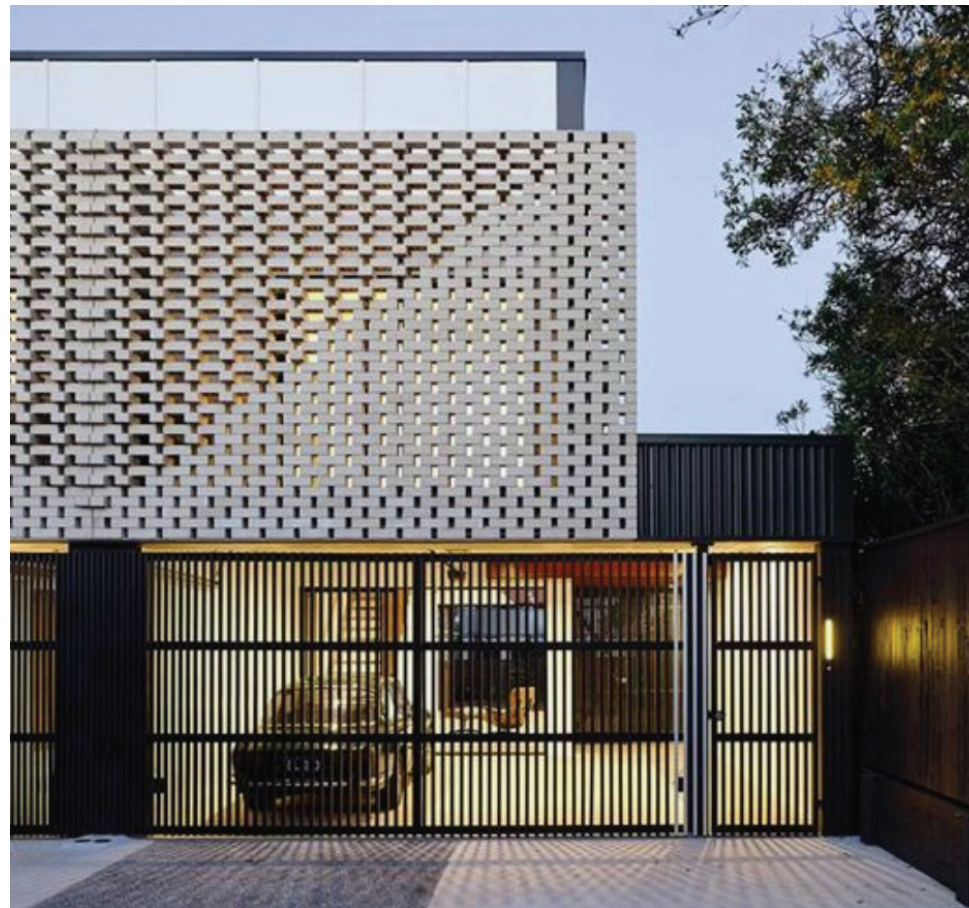
Perforated masonry brickwork
