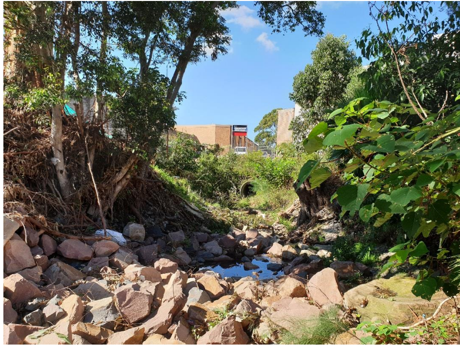
Photo B31: Inlet downstream of Winbourne Road
