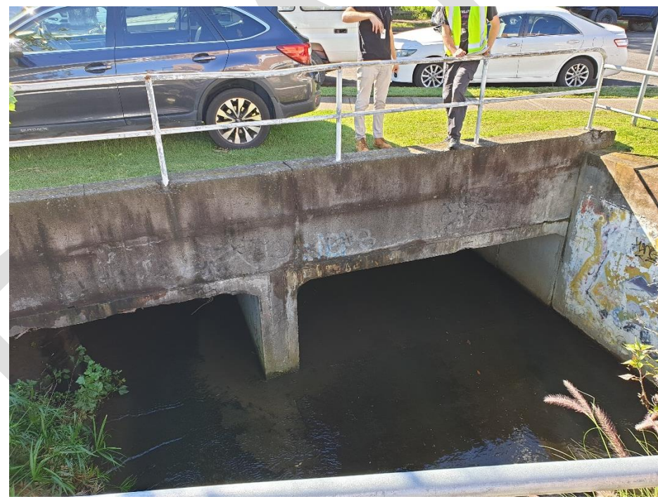
Photo B29: Culverts under Harbord Road
