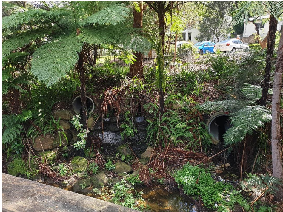
Photo B13: Outlets downstream of The Kilns
