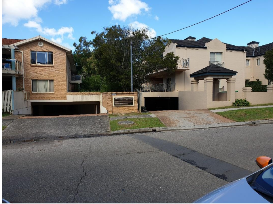
Photo B19: Properties downstream of Gulliver Street
