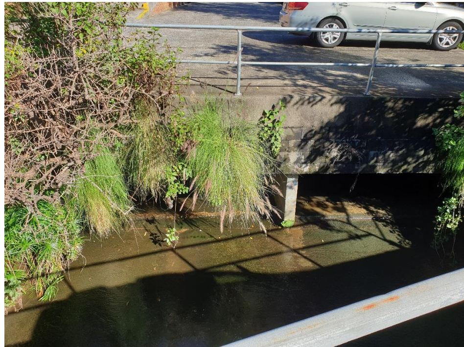
Photo B28: Culverts west of Harbord Road
