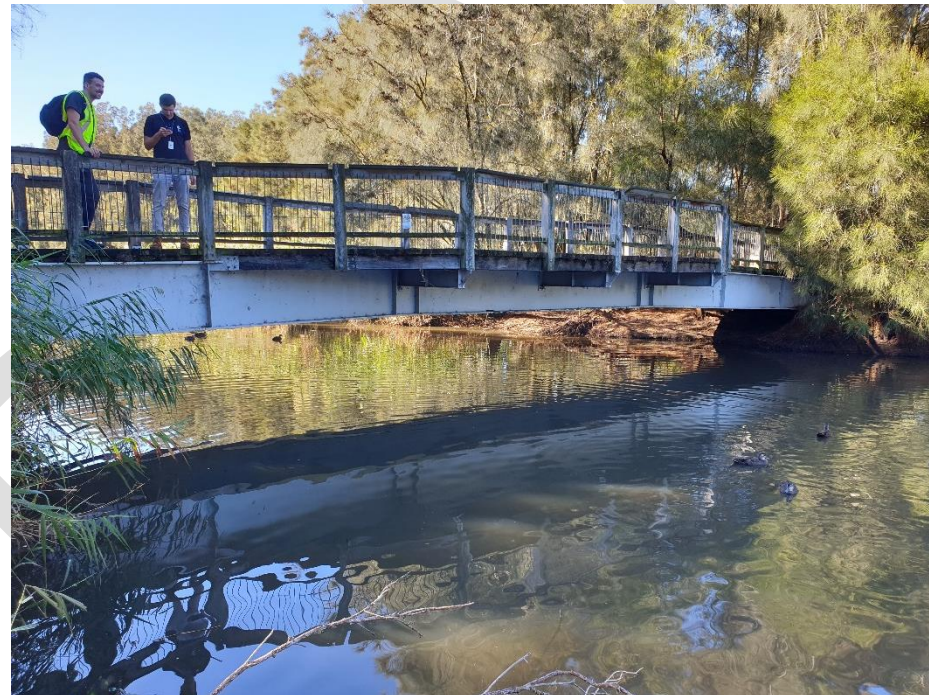
Photo B35: Eastern Pedestrian Bridge
