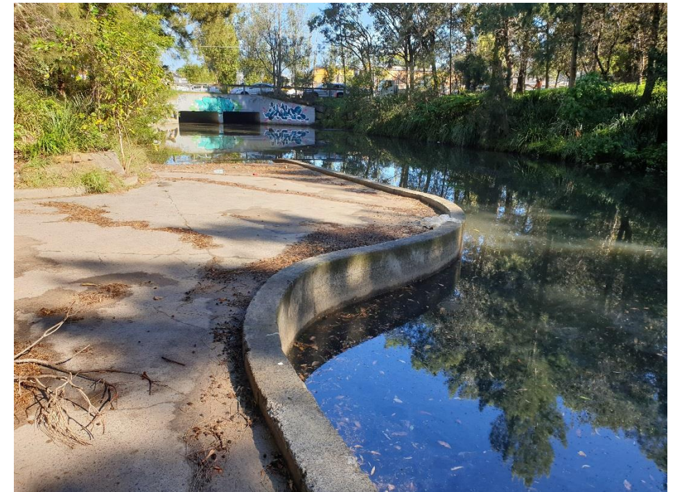
Photo B30: Downstream outlet from Harbord Road
