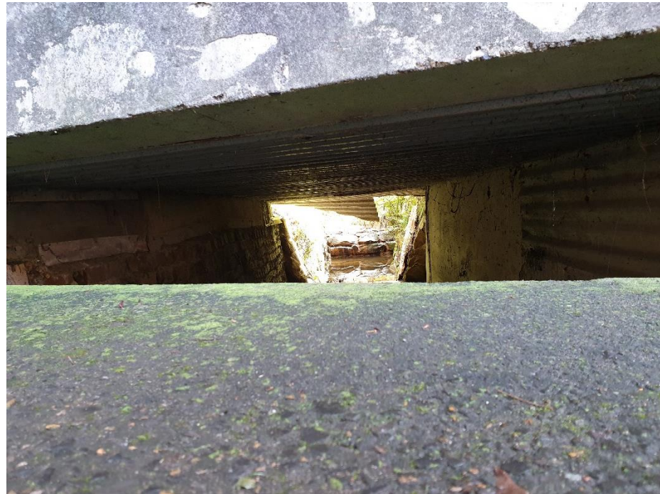
Photo B16: The Kilns Downstream Channel (Private Lane)
