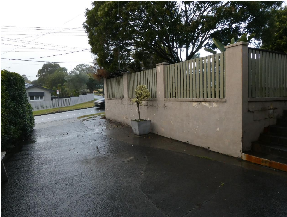
Figure 2: DRIVEWAY ACCESS FROM TRUMAN AVENUE
