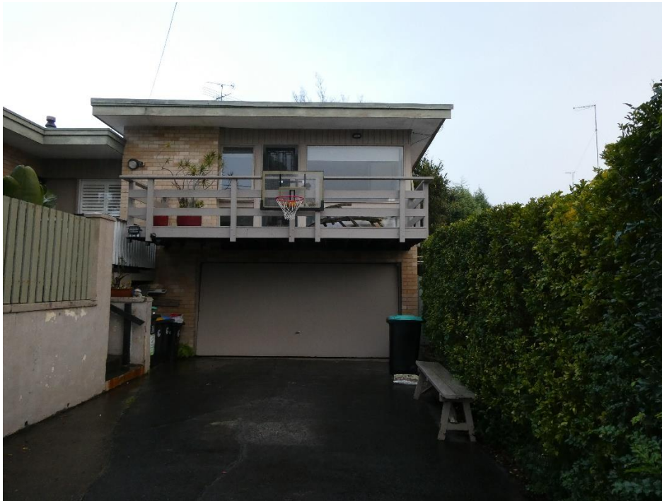
IMAGE 1: East side/front facade of property.
