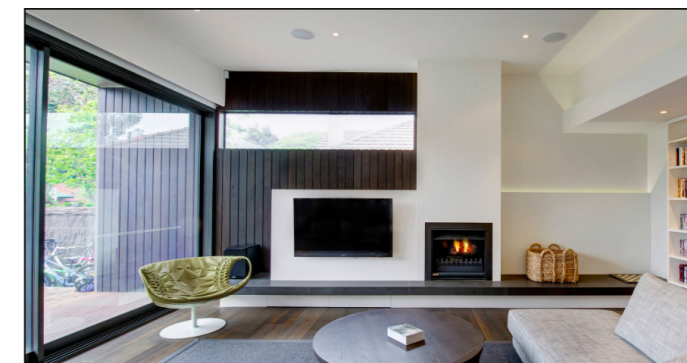
VTTP-01 VERTICAL TIMBER PANEL WITH PLASTER. POWDER COATED FINISH. WHERE MARKED ON ELEVATION.
