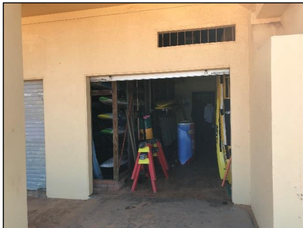
Figure 11. Storage areas with roll-up shutter doors. (Source: Heritage 21, 23.05.18)
