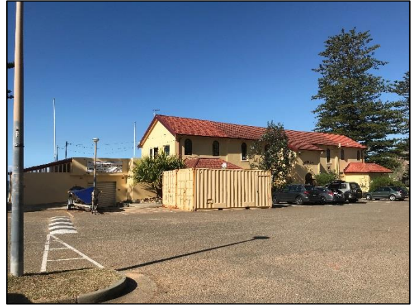
Figure 4. View from the north western corner of the parking lot looking towards the subject building. (Source: Heritage 21, 23.05.18)
