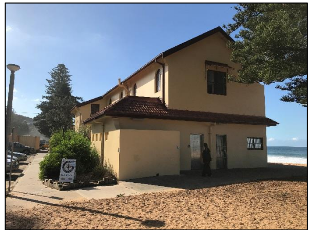
Figure 6. View of the southern wing and extension. (Source: Heritage 21, 23.05.18)
