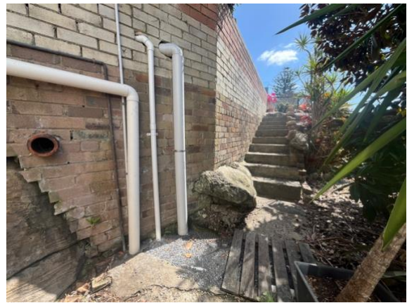
Photo 4: Brick wall in rear yard
