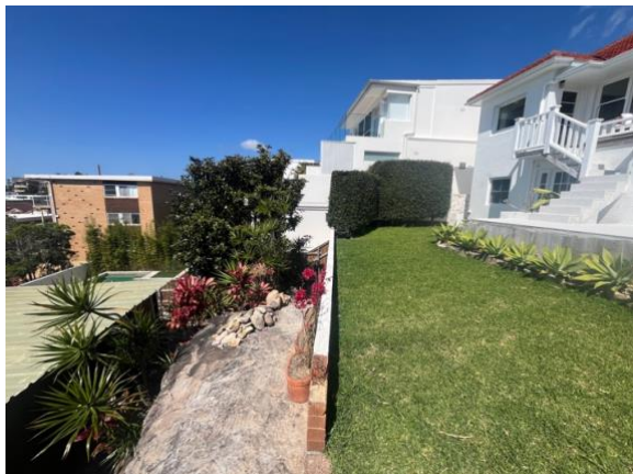
Photo 3: Brick wall partially over bedrock in rear yard
