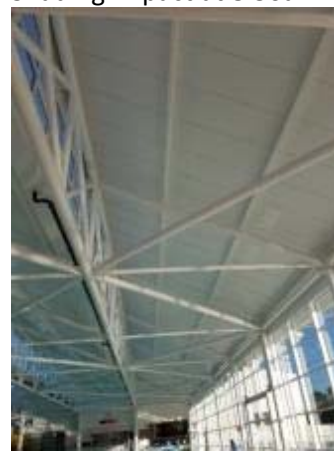
Internal roof structure
