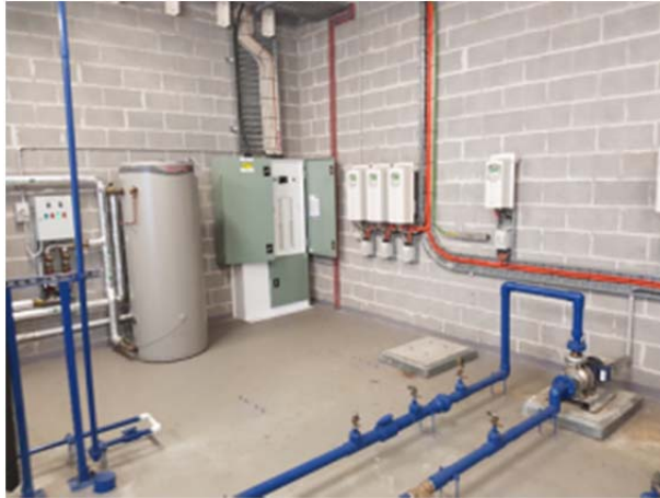
Main switch room
