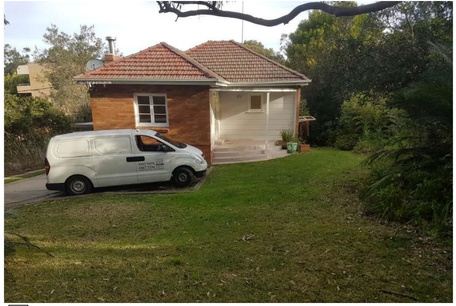
12 PROPOSED SITE EXISTING BUILDING 3 CENTRAL RD -
