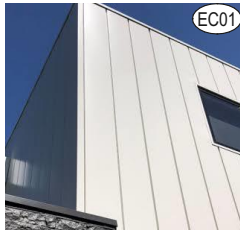
WHITE METAL CLADDING
