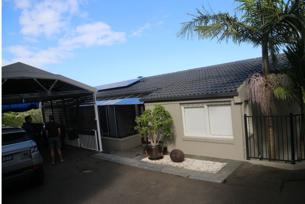
Figure 2.5 Current carport structure and associated dwelling house
