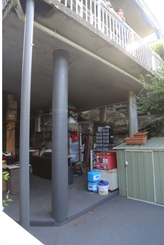
Figure 2.7 Undercroft storage area below the suspended concrete slab and carport.
