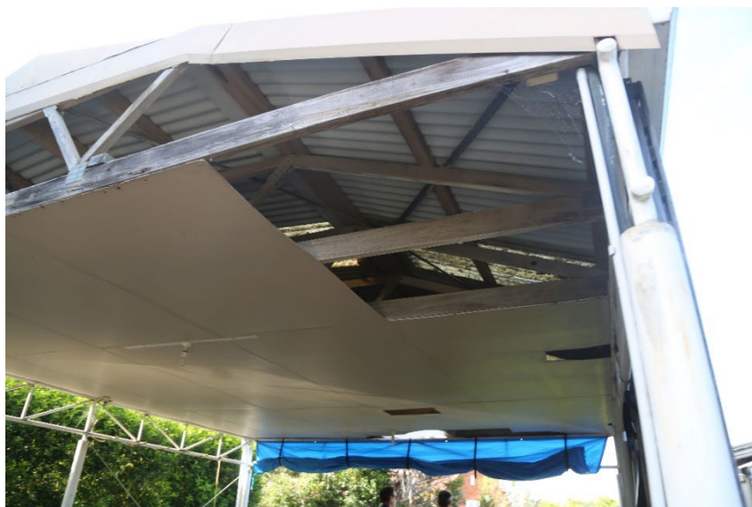
Figure 2.3 Current carport structure to be reconstructed as a garage
