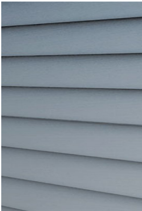
NEW WB / EX WB WEATHRBOARD CLADDING TO MATCH EXISITNG LIGHT GREY PAINT FINISH
