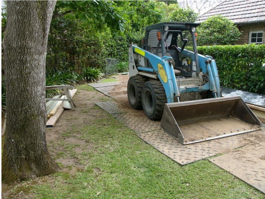
Figure 6 – Showing typical detail for truck mats.
