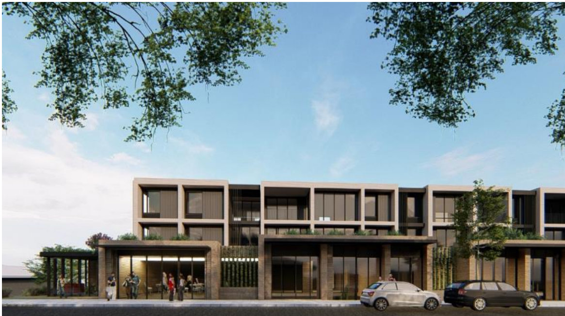
FIGURE 6: PHOTOMONTAGE – THE PROPOSAL VIEWED FROM LOCKWOOD AVENUE - DEMONSTRATING RECESSIVE NATURE OF UPPER LEVEL
