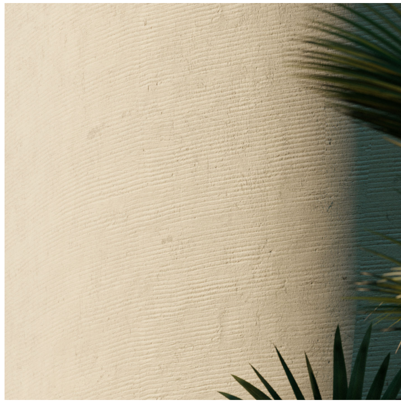
REN-01 - NATURAL LIME AND CEMENT RENDER (GROOVED FINISH)
