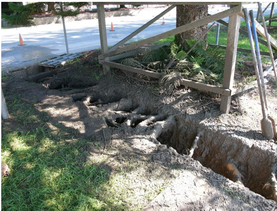
Figure 8 - showing completed trench with surface roots retained intact.
