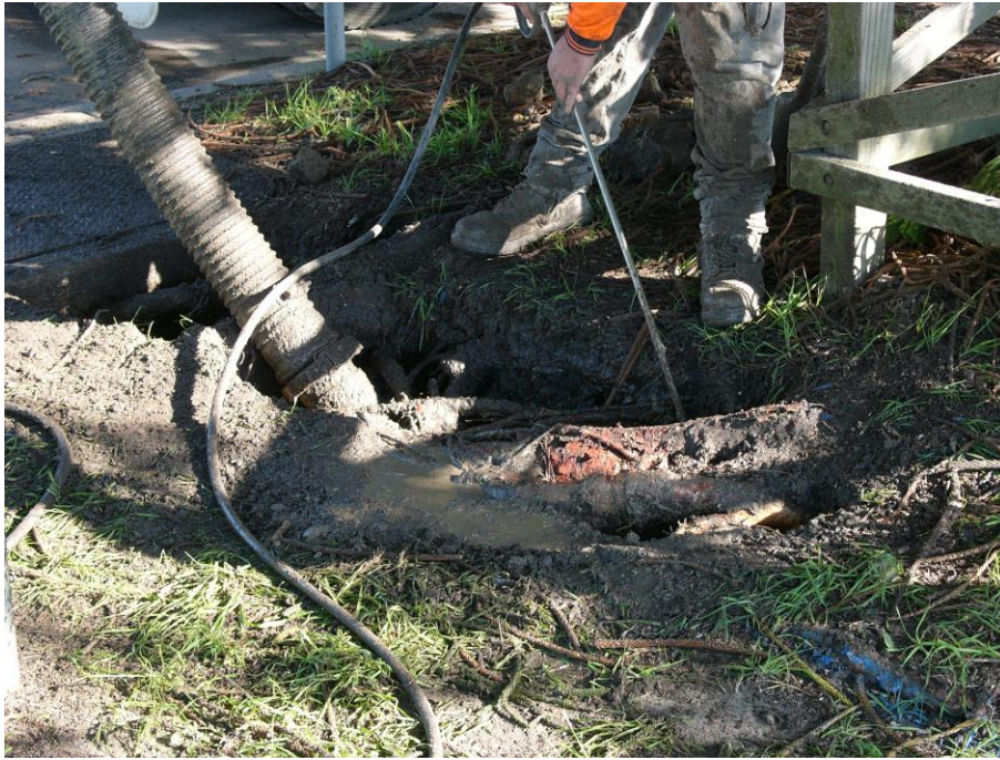
Figure 7 - showing excavation being undertaken using non-destructive excavation techniques (high pressure water lance with vacuum extraction unit).
