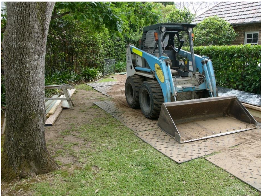
Figure 4 – Showing typical detail for truck mats.
