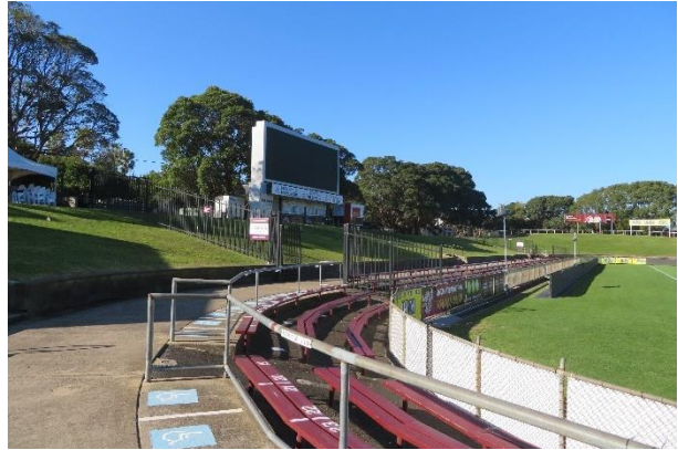
Figure 35 – Detail of bar on the northern Oval boundary topped by a screen.
