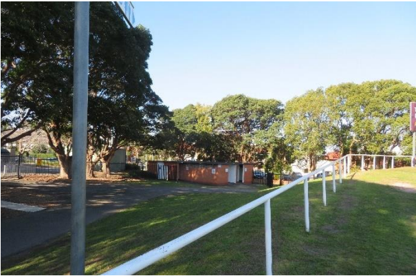
Figure 18 – View north east showing the tree plantings surrounding the toilet block. The entrance to the pre-school can be seen behind the fence.
