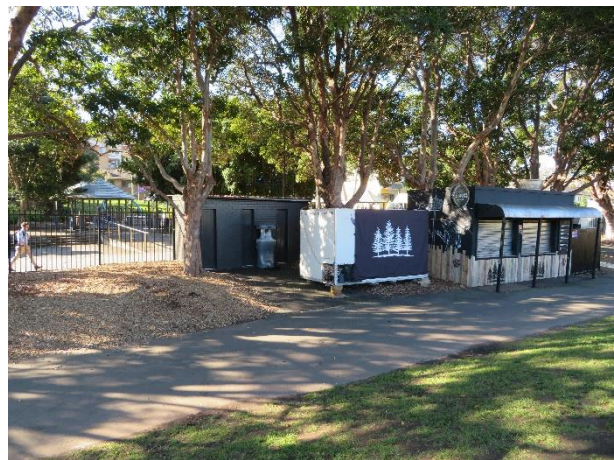
Figure 33 – Detail of the kiosk buildings along the northern boundary.
