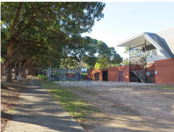
Figure 36 – View north of the structure on the western boundary behind the basketball and cricket facilities.
