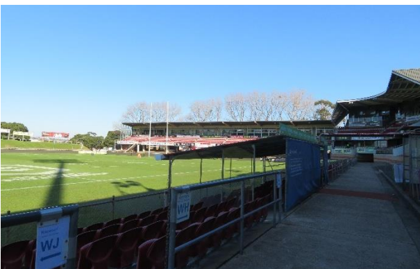
Figure 26 – View south showing the southern portion of the subject site.
