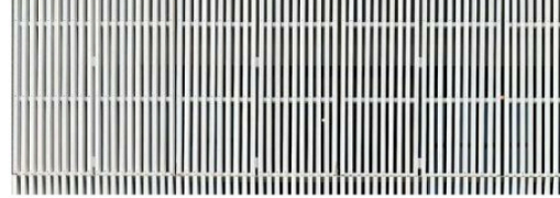
02 - SCREENING Angled aluminium batten white finish [scr01]
