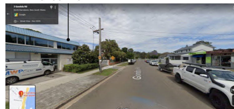
FROM SITE LOOKING TO THE WEST
