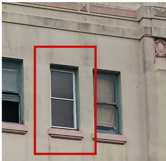
Reconstruct window to match original detailing.
