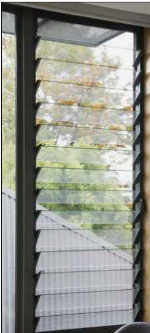
example of black satin powder-coated adjustable glass louvre window
