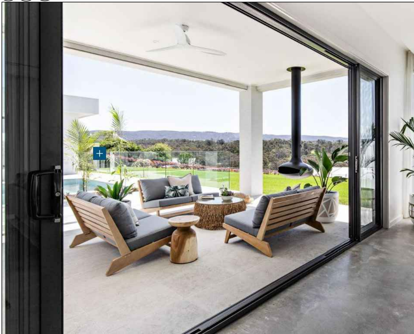
example of stacked sliding black satin powdercoated aluminium framed glass doors concept ie between new enclosed space on balcony and open balcony space. Showing full open corner scenario proposed
