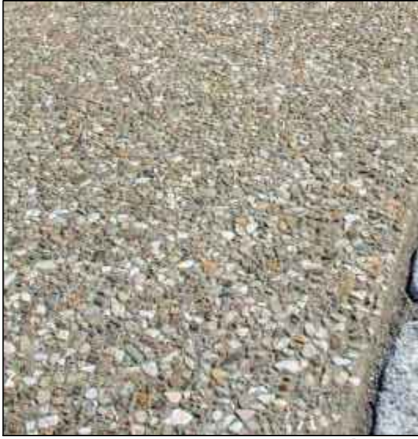
rc slab with washed aggregate finish to new paved area on north side of building
