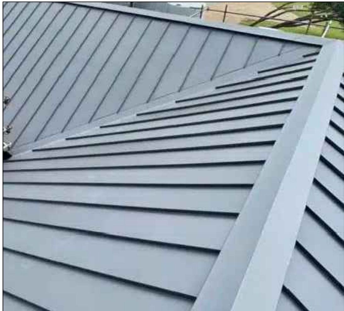
proposed raised seam metal deck roofing in light grey colour sim 'Shale Grey' Colorbond
