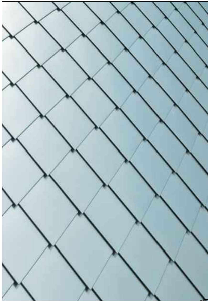
proposed rhomboid shaped shingle 'scales' patterned cladding. Colour proposed is mixture of Selector Steel Unicote Extreme colours shown here
