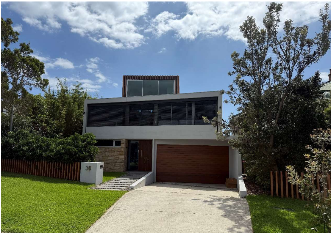
Figure 3 – A three storey dwelling at 30 Hillcrest Avenue Source: NBP
