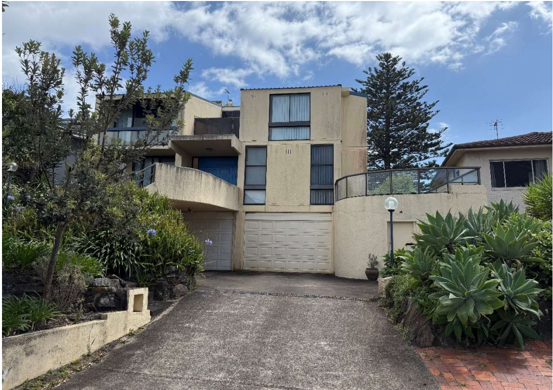
Figure 4 – A three storey dwelling at 16 Hillcrest Avenue Source: NBP
