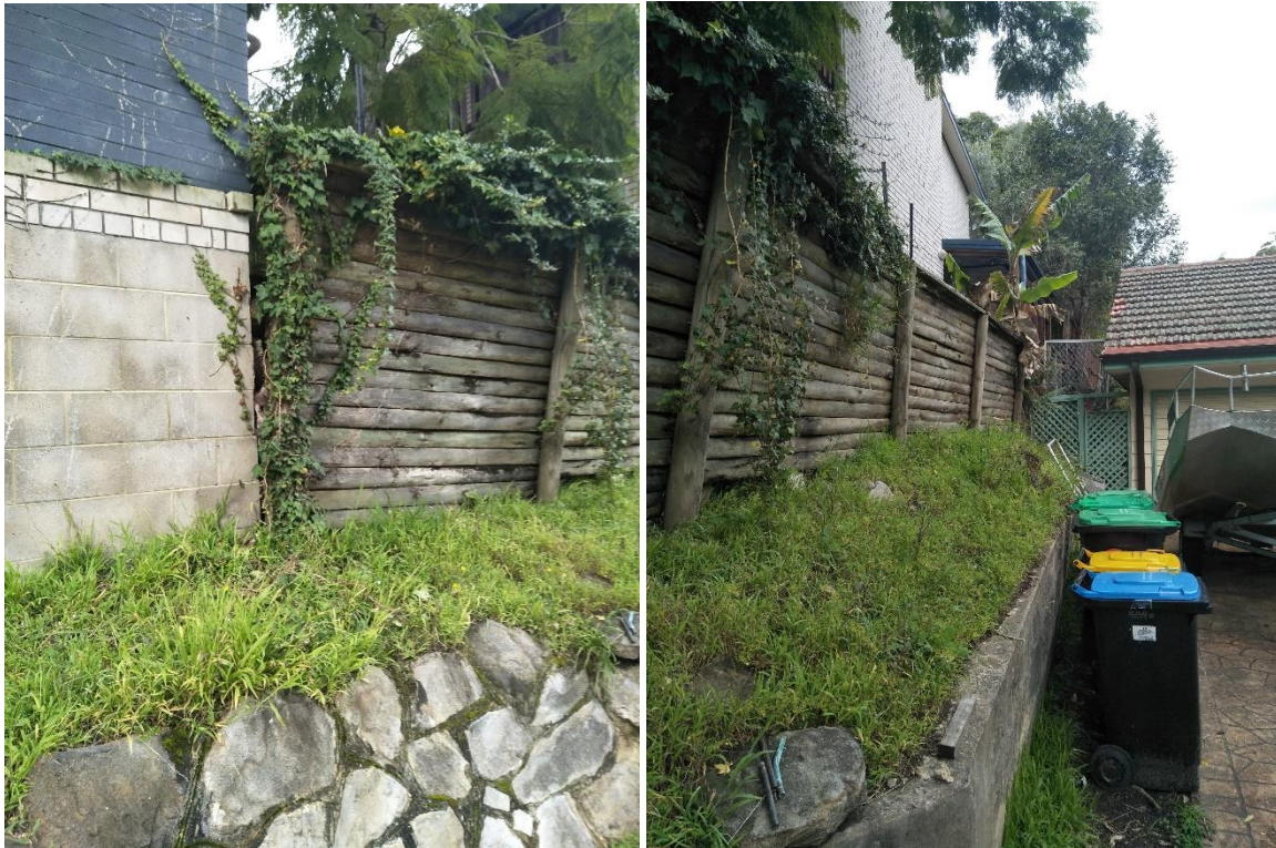
Photos of existing retaining wall to be demolished and replaced with new engineered retaining wall
